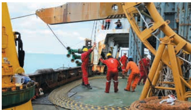
Activities on board during the Batam-Dumai-Melaka (BDM) submarine cable project.
