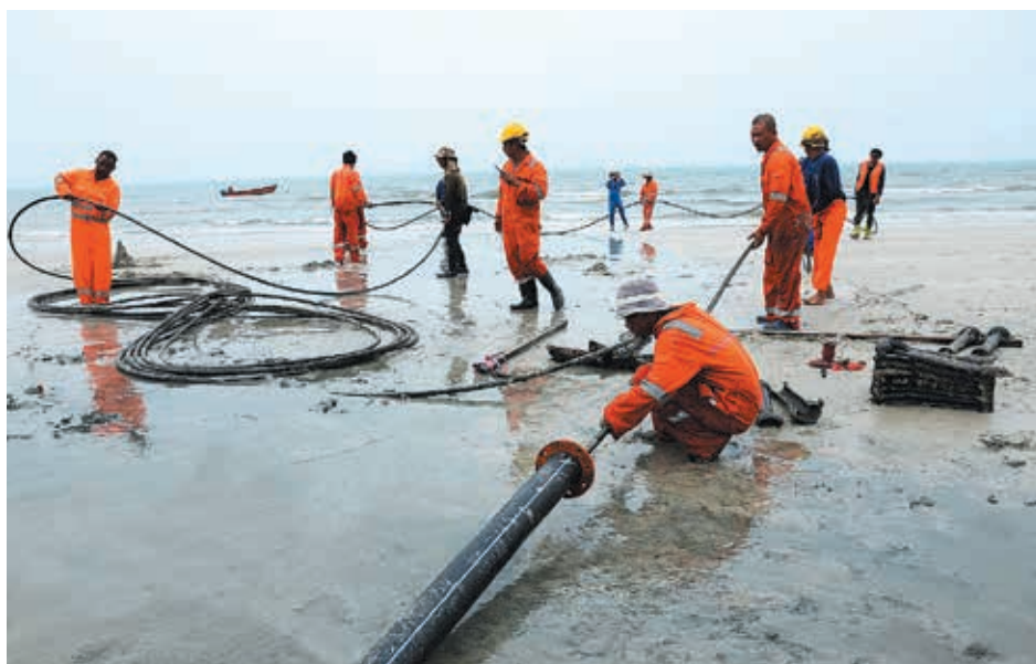
Beach works of the newly-landed Cahaya Malaysia (CM) submarine cable towards TM Mersing cable landing station.
