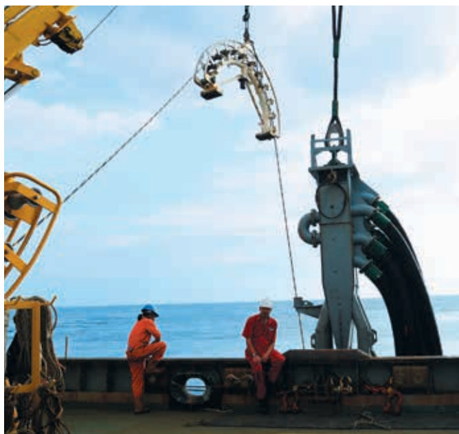
Installing the last stretch of cable for Batam-Dumai-Melaka (BDM) submarine cable system.
