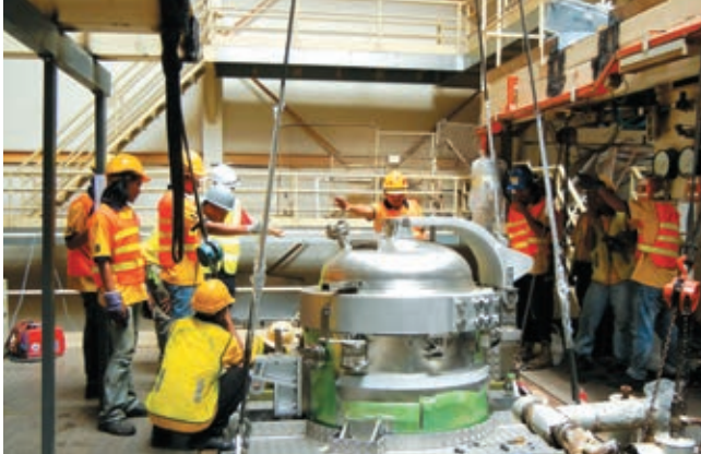
Upgrading of the Dry Ice Expanded Tobacco Plant was conducted from October to December 2012.
